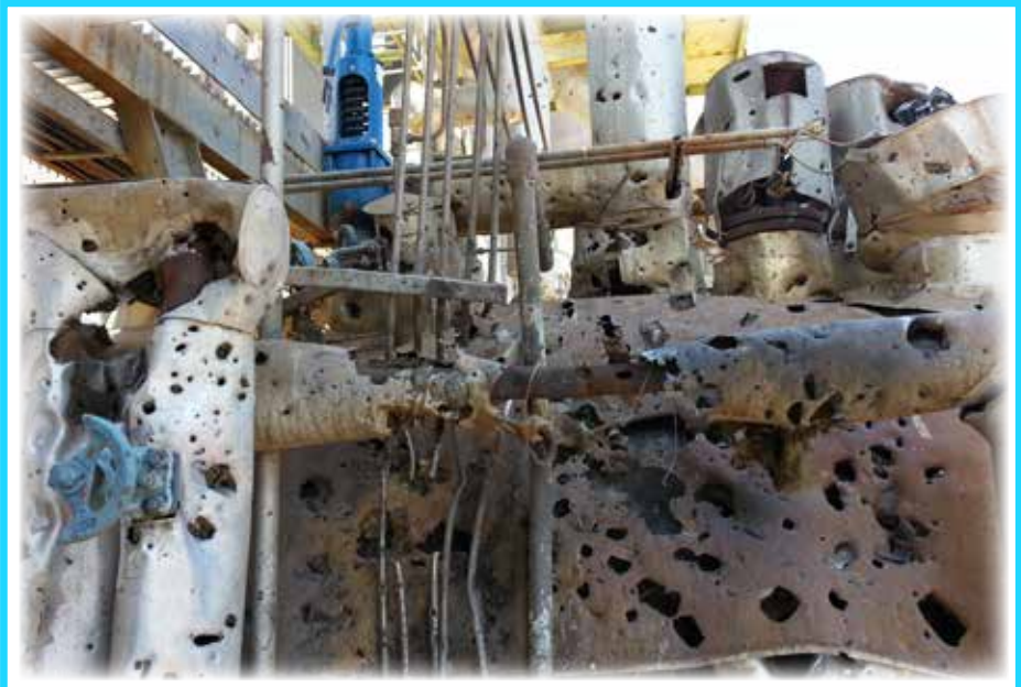
Damage to power plant machinery
