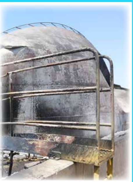
Fuel tanks destroyed
